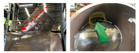
Fig.2. (a) The location of the inner weld direction on the node from an external perspective. (b) The location of the inner weld direction on the node from an internal perspective. The welder must overcome the narrow space and angle limitations.
